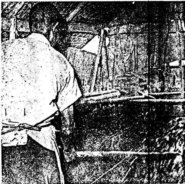
Above, the sieve-bend grizzly. Underflow launder in foreground handling 3,000 g.p.m. Bar spacing set to reject plus \frac{1}{2} -in. Swing deflector board, level with author's right hand, prevents loss of near-oversize by bouncing
